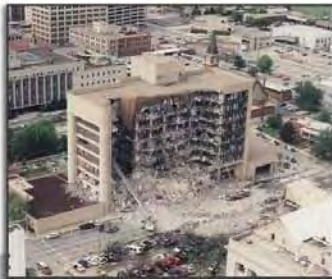
Murrah Building, Oklahoma City April 26, 1995
